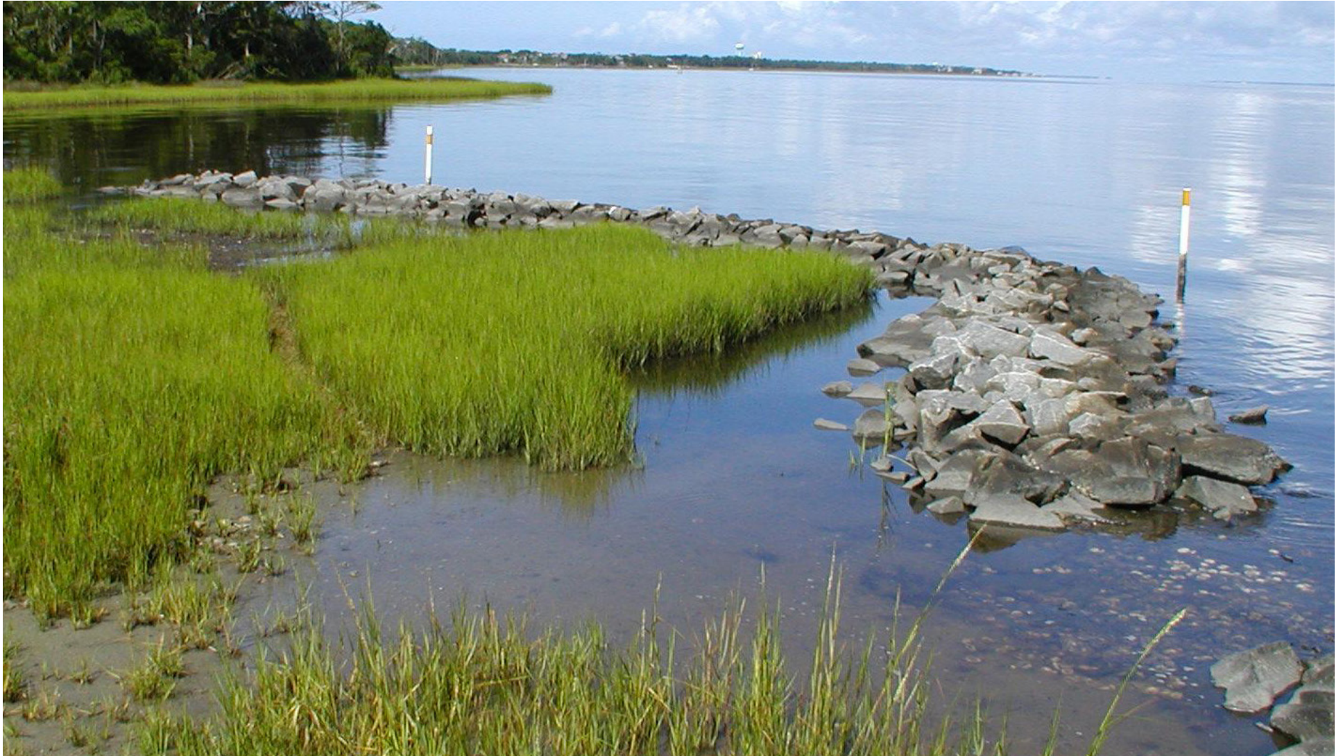
Living shoreline constructed in 2001
