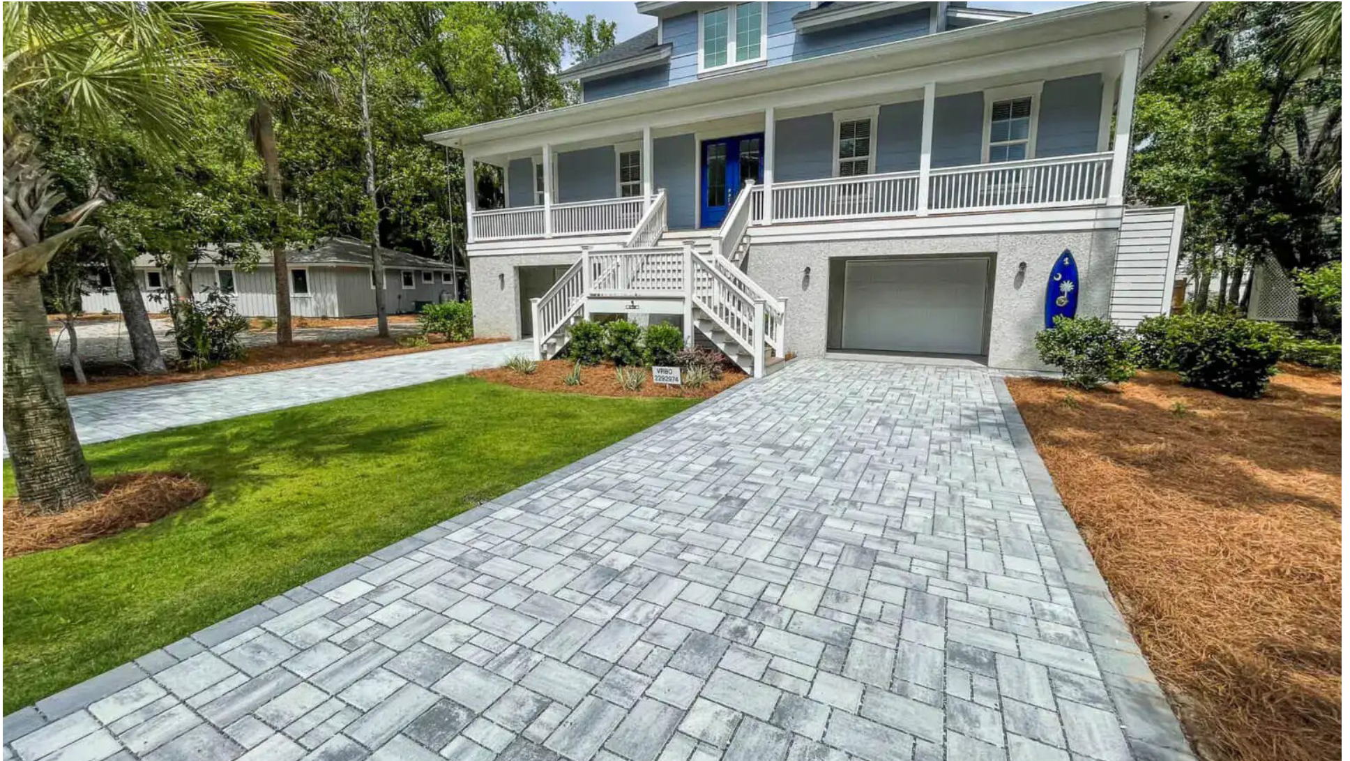
Permeable Paver Driveway in South Carolina Credit: American Paving Design
